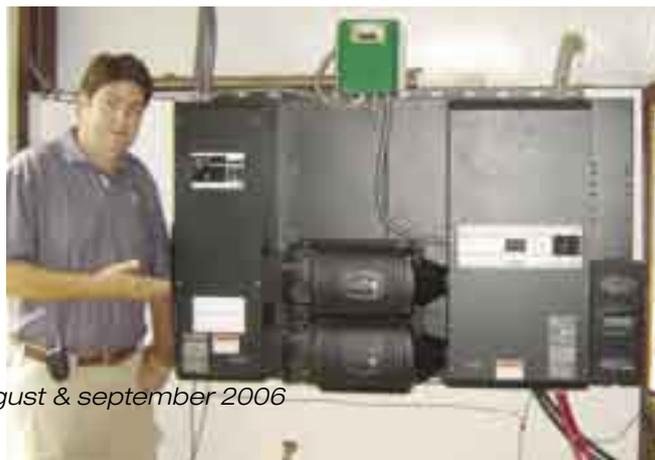
system monitor, and OutBack disconnects all prewired. This UL-approved power panel supplied by Conergy Inc. simplified the installation and can accommodate up to four inverters if needed. Phil Undercuffler at Conergy and Matt Rust at OutBack were very helpful in the design of this panel, and Conergy had it built and shipped in two days!
